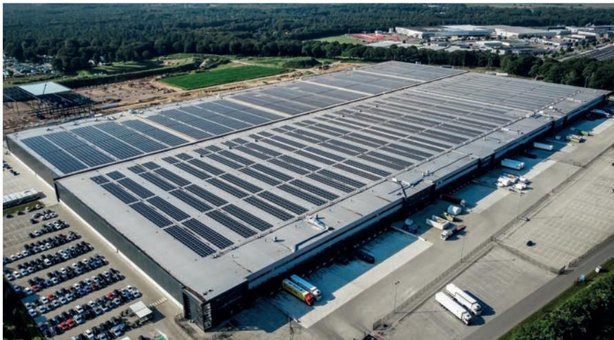
Photovoltaic plant in Gennep, The Netherlands
